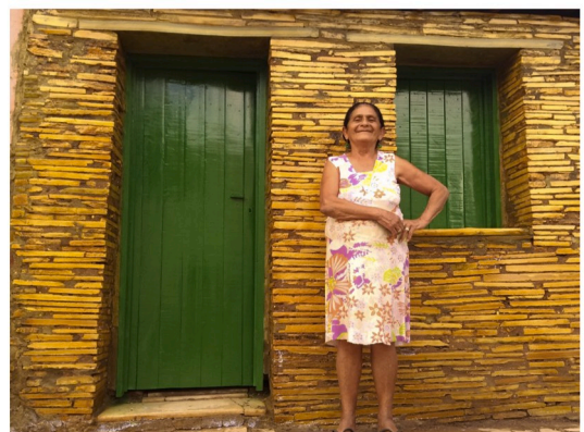
Fig. 12. The restoration of the Inhumas houses by replacing the old coating (A) by the local Cairiri Stone (B).
