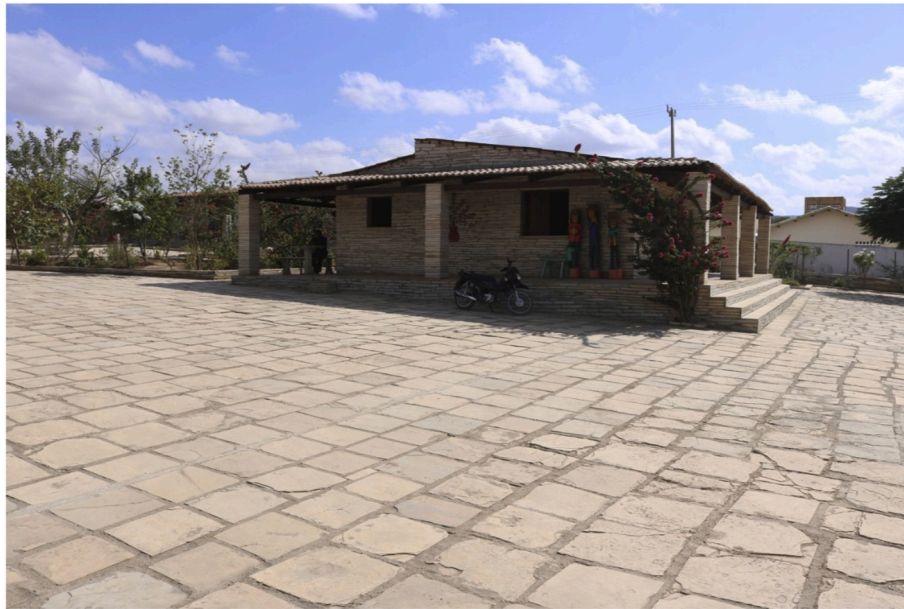
Fig. 5. The entire infrastructure of the Casa da Pedra was built with Cariri Stone exploration waste, which had already fallen into disuse. The construction of the Casa da Pedra and the planting of vegetation, particularly species typical of the Brazilian backlands (“sertão”), followed the recovery of the traditional methods in the region.
